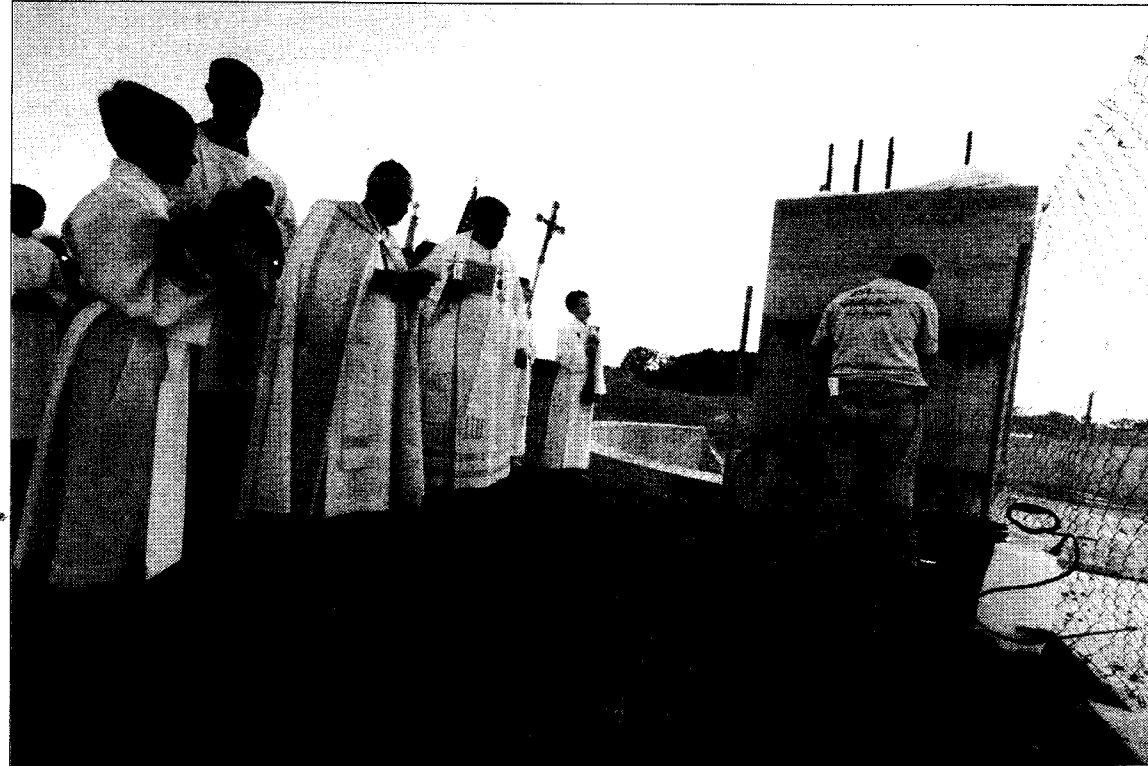
Cardinal George and Father John Jamnicky (right) watch as Anthony Fernandez of JSL Masonry Restoration seals the cornerstone during the blessing and laying of the cornerstone for St. Raphael the Archangel Church on Sept. 29 in Old Mill Creek. The church is using pieces of closed churches in its construction. Right, Cardinal George signs a document that was to be sealed in a time capsule and placed in the church foundation.
